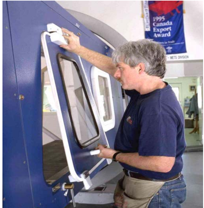
Escape Exit Installation
